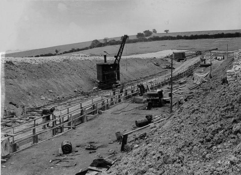
2. Down Stream face of Dam nearing completion. Tail bay in Foreground. 5.6.39. 3. Tail Bay in course of construction. 3.10.38. 4. Northern end of Puddle Trench, showing lights, so work could be continued at night. 29.7.38.
